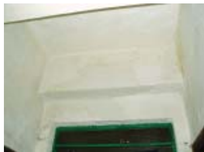
Ceiling water leakage
